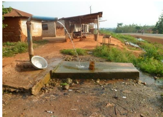
Picture 2: Simple artesian borehole at Gbefagie
