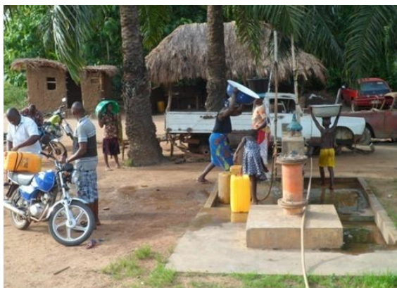
Picture 1: Artesian boreholes with a tap at Atchabita
